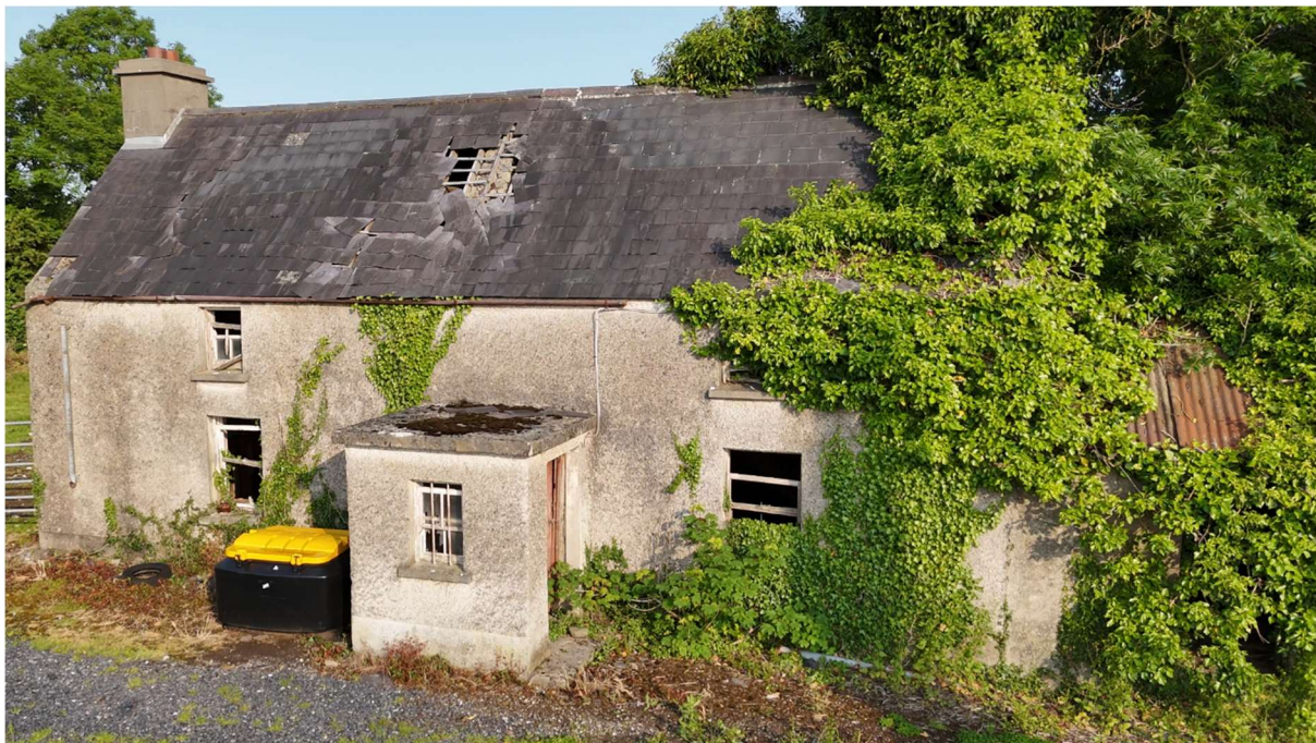
Figure 2.5 Photograph of derelict dwelling to be demolished
